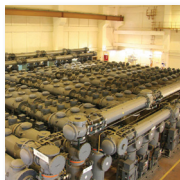
400kV Gas Insulated Switchgear
