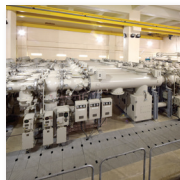
275kV Gas Insulated Switchgear
